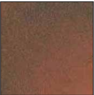
M9 - CORRODED COPPER
