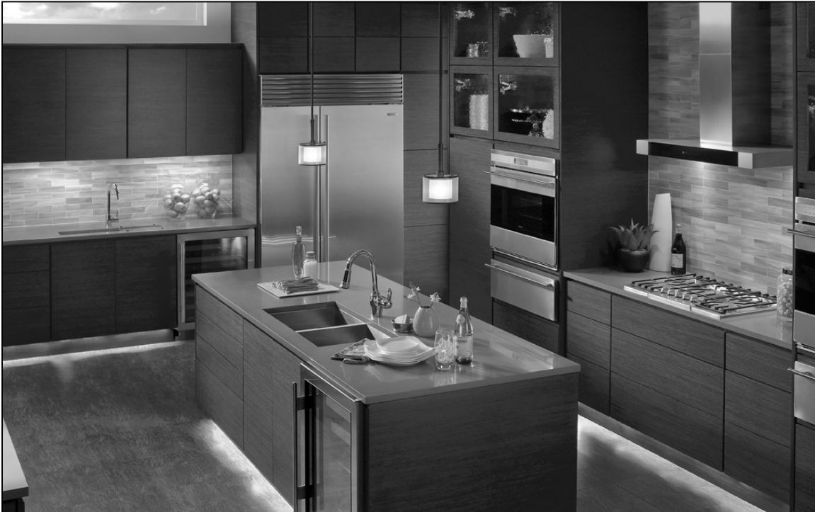
Kitchen with undercabinet, over cabinet and toekick lighting along with overhead pendant accent lights. Exhaust fan carries its own lights and glass front cabinets all have a light inside, but are turned off in this photo.
